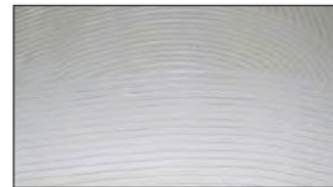
Example of properly troweled adhesive application
