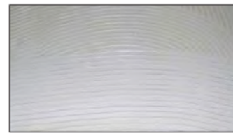
Example of properly troweled adhesive application
