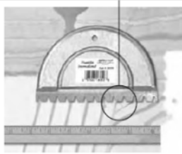
Example of properly troweled adhesive application
